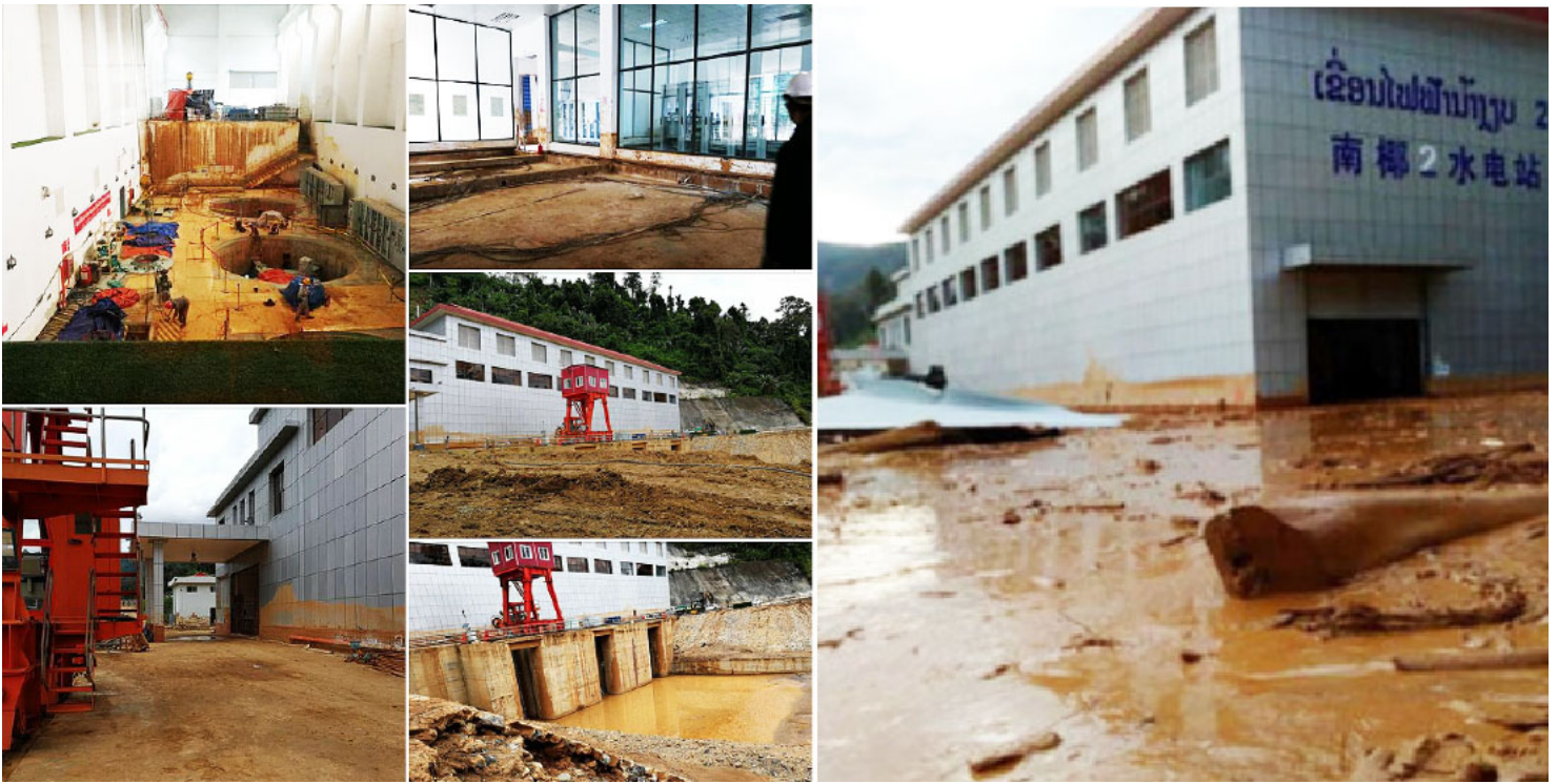
Nam Ngiep 2 powerhouse image below:
